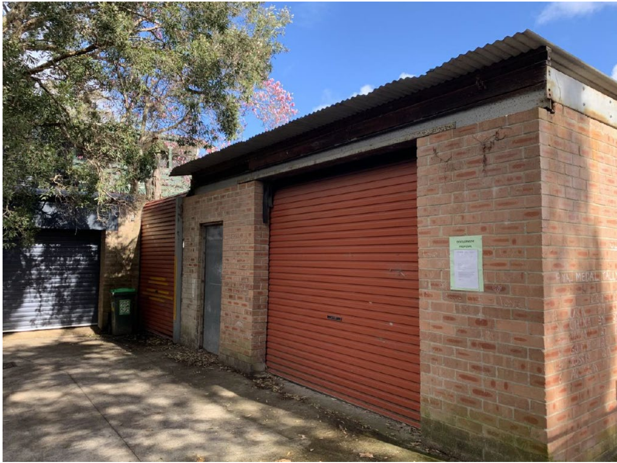
Site viewed from Kingsclear Road
